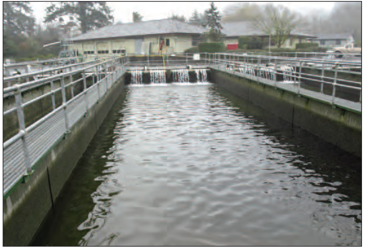
A new, improved weir at the Salmon River Hatchery will ensure a reliable supply of water and help the hatchery meet its goals for producing salmon, steelhead and trout.
