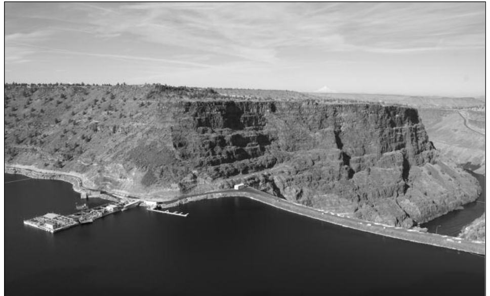
Lake Billy Chinook is formed by Round Butte Dam constructed at the confluence of the Deschutes, Crooked and Metolius rivers. The Selective Water Withdrawal facility is visible on the left. Photo by Jim Yuskavitch
